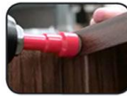
Step 5 : Take drill with screw holder and fit fence Stainless Steel screw into the holder. Securely fix screw through Top Panel and Post Cover joining them as shown.
