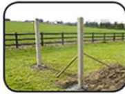
Step 1 : Secure your structural inner posts firmly on site.
