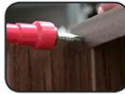
Step 5 : Take drill with screw holder and fit fence Stainless Steel screw into the holder. Securely fix screw through Top Panel and Post Cover joining them as shown.
