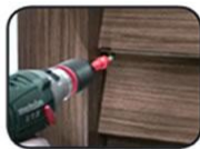
Step 7 : Once the Standard Panel is in position fix it securely to the Top Panel and Post Covers using the ball nosed Stainless Steel assembly screws provided as shown above. Follow this procedure for the next panels fitting them together.
