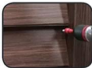
Step 7 : Once the Standard Panel is in position fix it securely to the Top Panel and Post Covers using the ball nosed Stainless Steel assembly screws provided as shown above. Follow this procedure for the next panels fitting them together.
